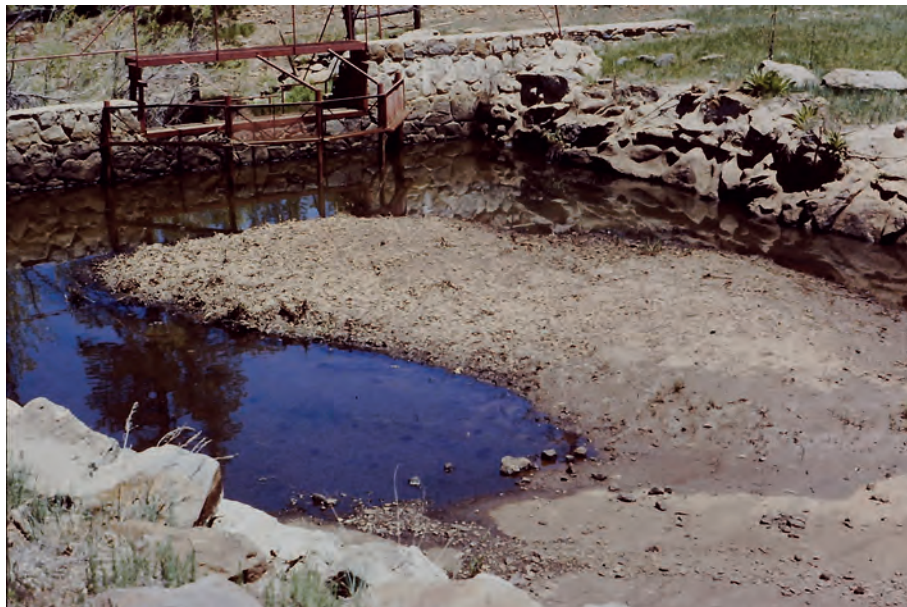
Figure 6.2. Deposition of bed load particles in a settling basin following the cessation of streamflow from a watershed (photograph by Peter F. Ffolliott).
