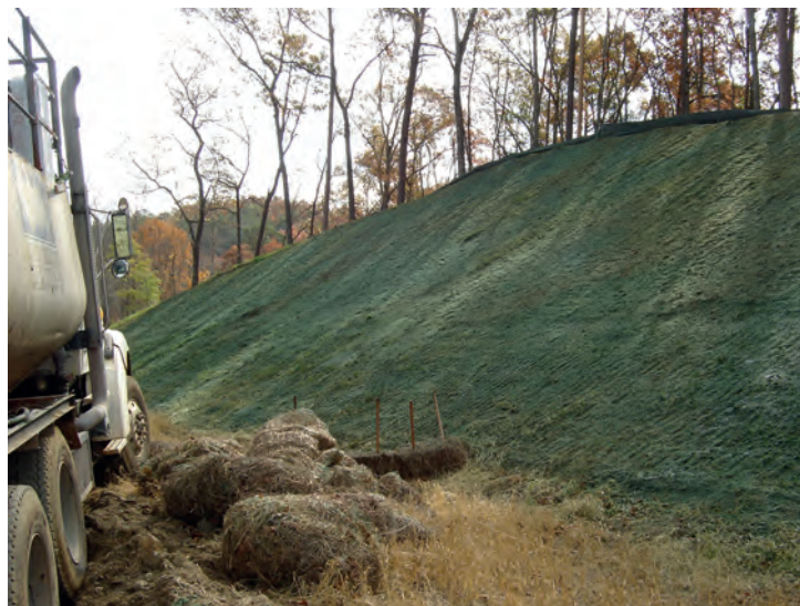
Figure 2.3. An eroding hillslope to be stabilized by establishing a vegetative cover by hydroseeding. The slurry applied to the site is often transported to the hillslope in a tank located on a truck (image from North American Green at www.nagreen.com ).
