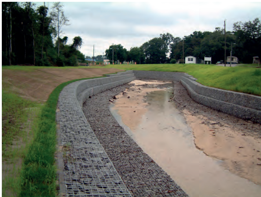
Figure 3.3. The side-slope of a stream channel is by gabion baskets. The gabions baskets form a retaining wall to stabilize a gully or stream channel to prevent further erosion (image from Modular Gabion Systems at www.gabions.new ).
